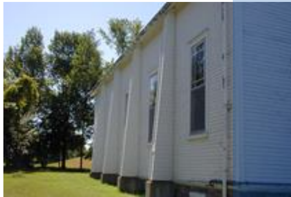
Photo of the added buttress supports.
