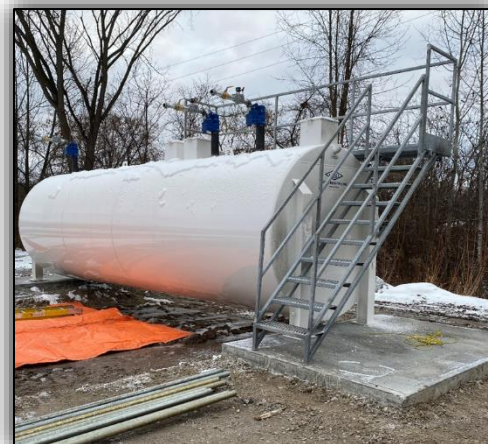
Above ground fuel tank during construction 2023
